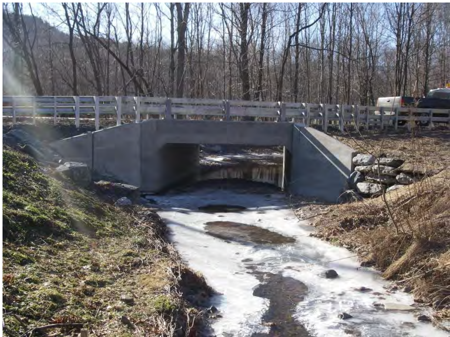
Figure 2.11 After restoration of an undersized and failing culvert in Lexington.
