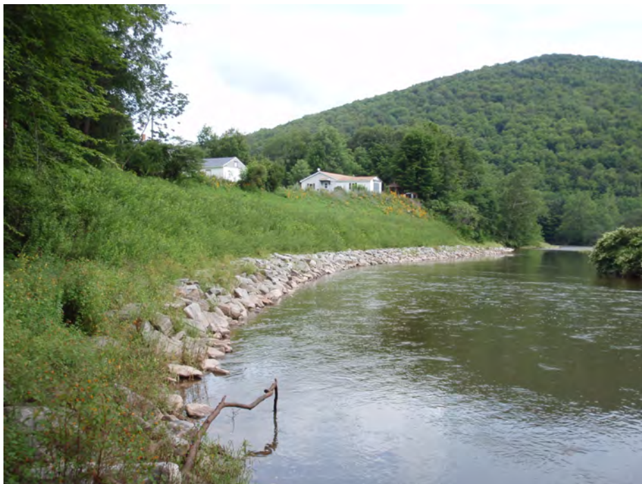
Figure 2.13 Terrace Avenue after streambank stabilization.
