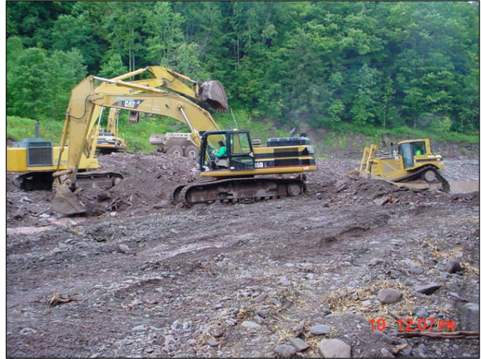
Phase I stream channel excavation.
