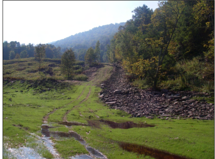
Stabilized borrow area access road and channel.
