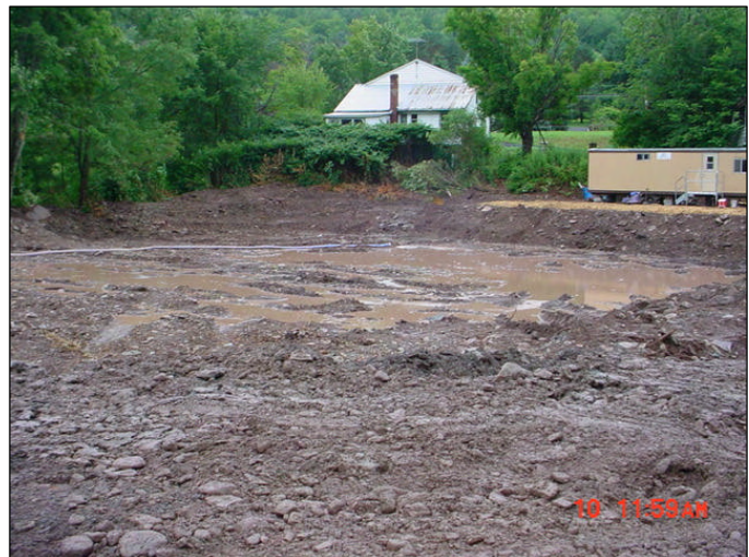
Phase I turbidity control basin.
