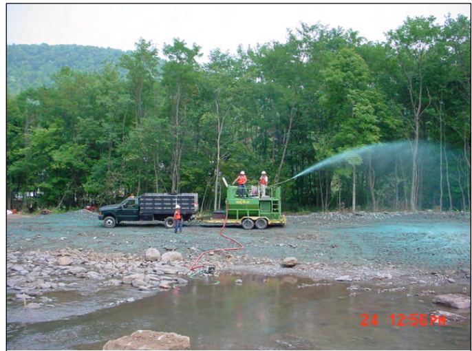
GCSWCD staff applying rye seed mix for initial vegetation establishment.
