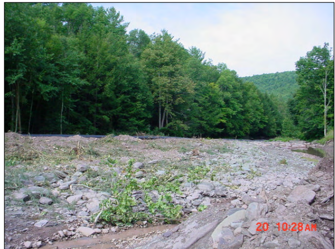
Clearing and grubbing of Phase II.
