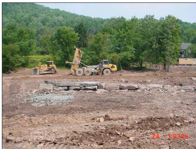
Completed arm of the downstream cross vane.
