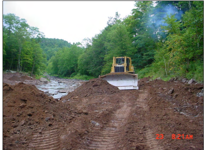
Final grading with topsoil material.
