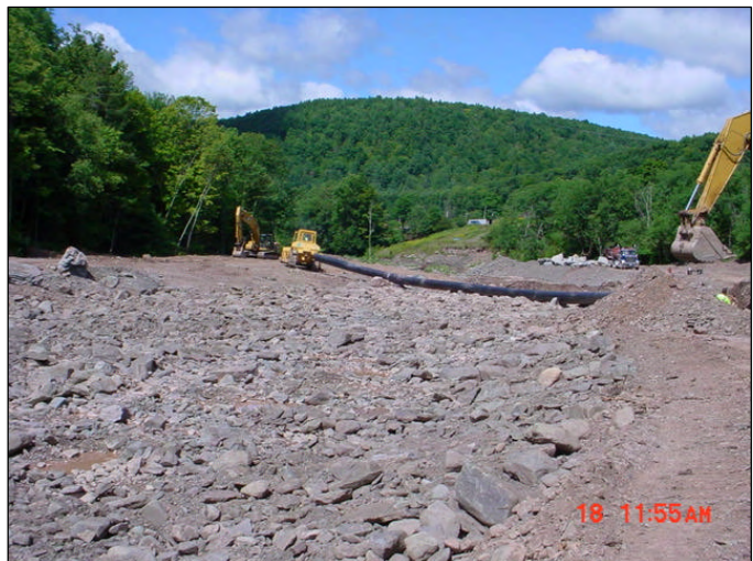
Section of the constructed riffle displaying salvaged and seeded coarser substrate.
