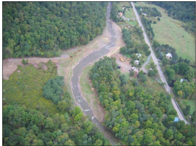
Aerial image of constructed condition taken September 2007.
