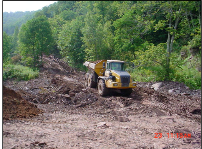
Off road truck delivering materials from the on-site borrow area.
