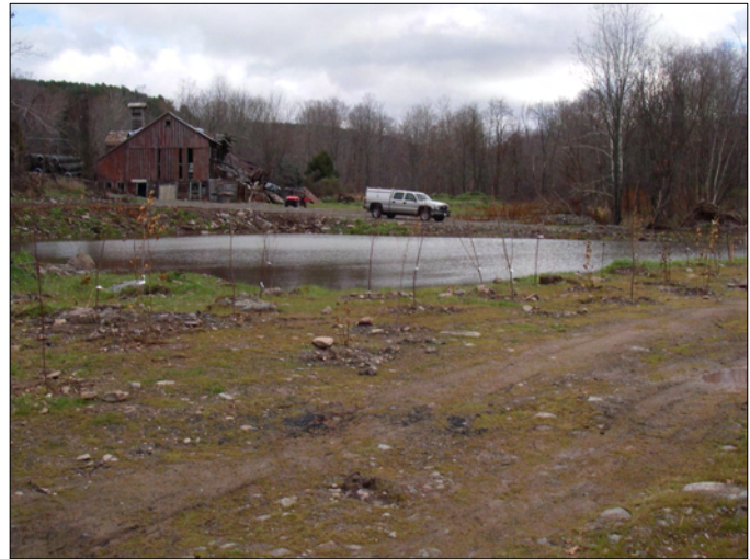
Constructed wetland mitigation area after a rainfall event.
