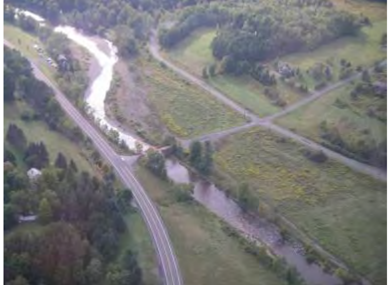
Figure 1. Aerial view of Carr Road project reach. Project is located to the right of the Schoharie Creek in the above photograph.
