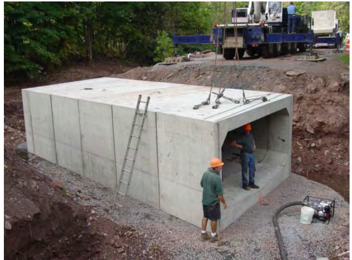
Photo 8: Culvert sections being set and leveled on tamped stone base,
