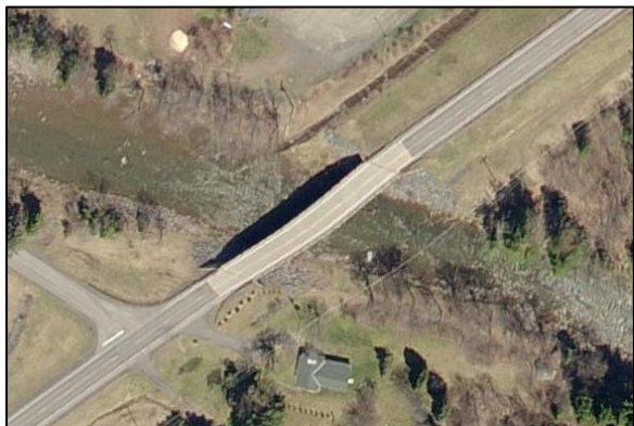
NYS Route 214 bridge at Station 119600
