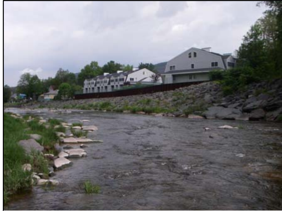
Melody Woods Complex 2006 (Station 109900-109350)
