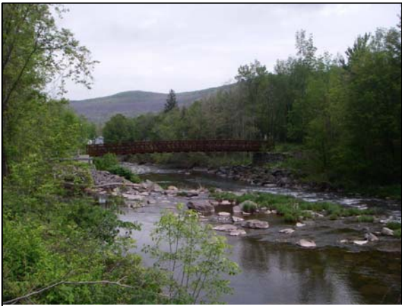
Foot bridge at Station 110470
