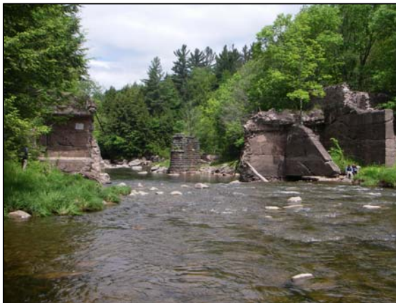
Old dam at Station 123240
