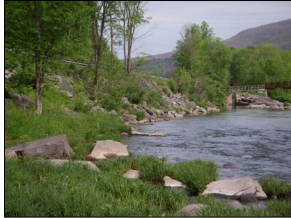
Rip-rap at Station 111140
