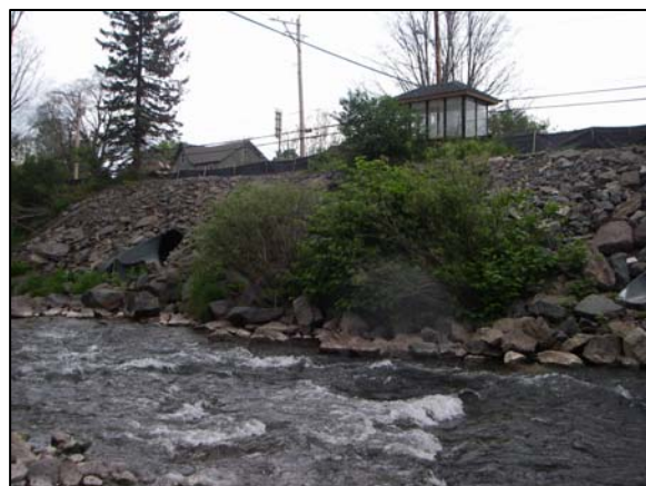
Rip-rap at Station 108500
