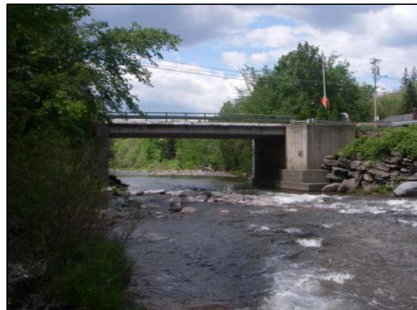
Bridge at Bridge Street – Station 104521
