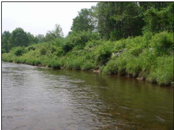
Rip-rap at Station 92040
