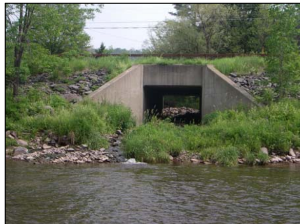
Tributary at Station 97500 - looking upstream
