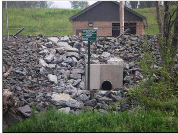
SPDES outfall at Station 98300
