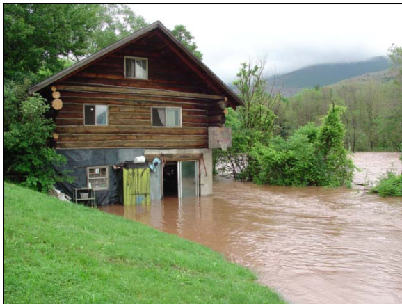
Flooding of residence at Station 84700
