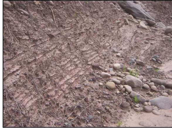
Clay exposure at Station 88900
