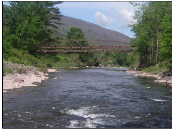
Bridge at Carr Road (Station 83957)
