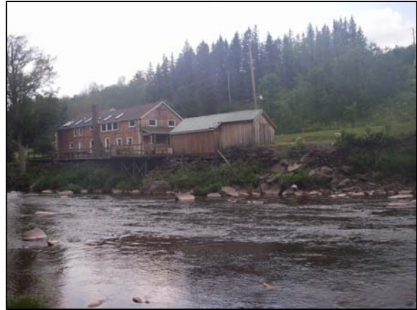
Stacked rock wall at Station 86250
