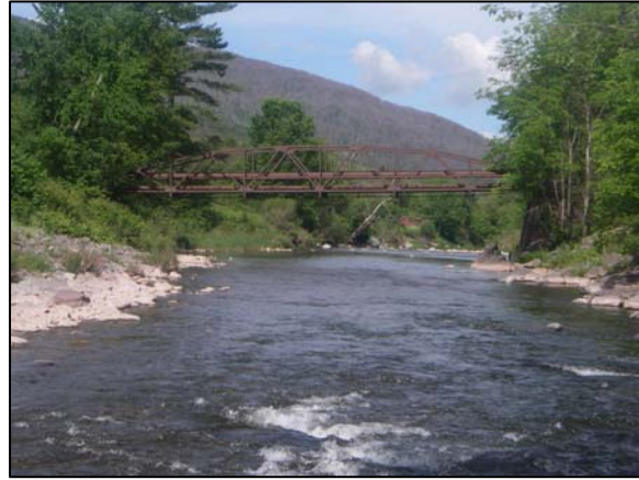
Bridge at Carr Road (Station 83957)
