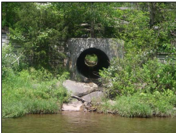
Culvert and Tributary at Station 80800
