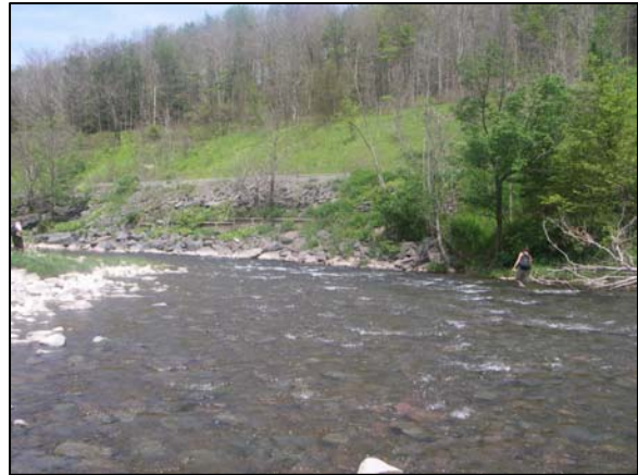
Revetment at Station 82300
