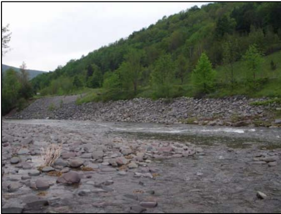
Rip-rap at Station 65200
