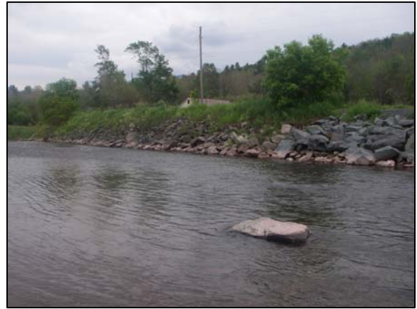
Rip-rap at Station 68300
