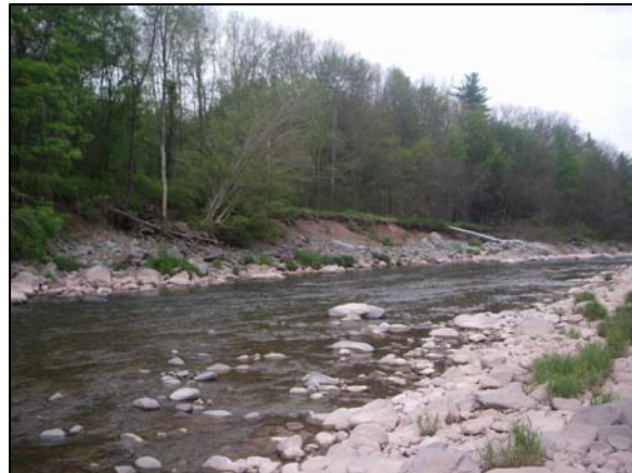
Bank erosion at Station 70450
