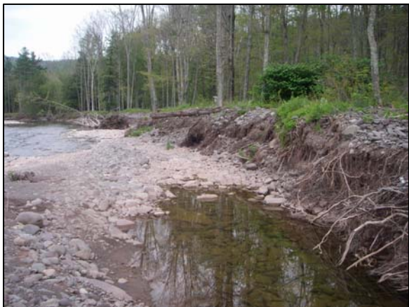
Bank erosion at Station 68900
