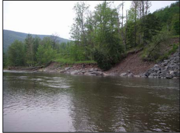
Bank erosion at Station 64580
