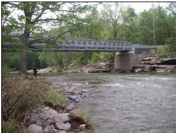
Bridge at Bush Road Station 63446
