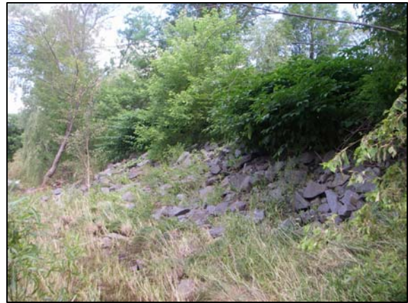
Rip-rap at Station 56600
