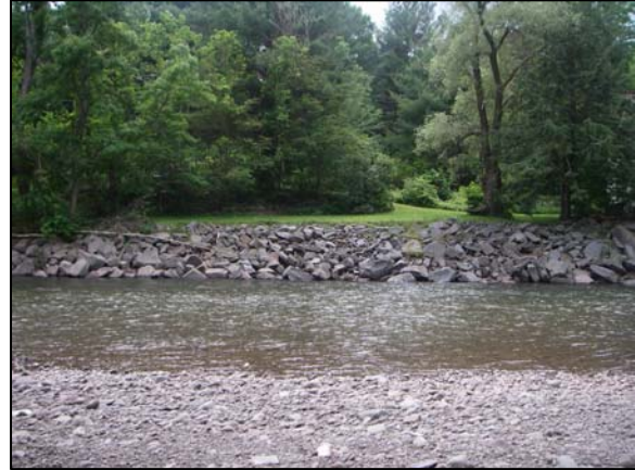
Rip-rap at Station 52120
