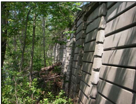
T-wall at Station 49450
