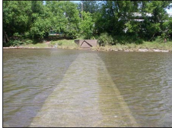
Concrete sill at Station 54480
