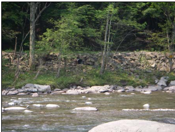
Rip-rap at Station 42050
