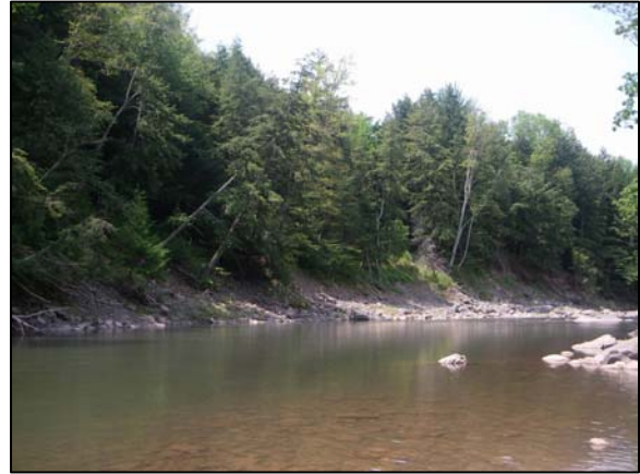
Bank erosion at Station 46750
