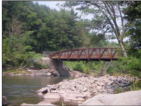
Mosquito Point bridge at Station 41722
