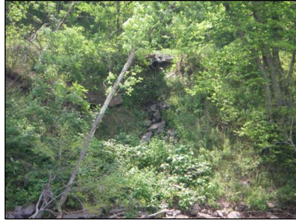
Stormwater outfall at Station 36350
