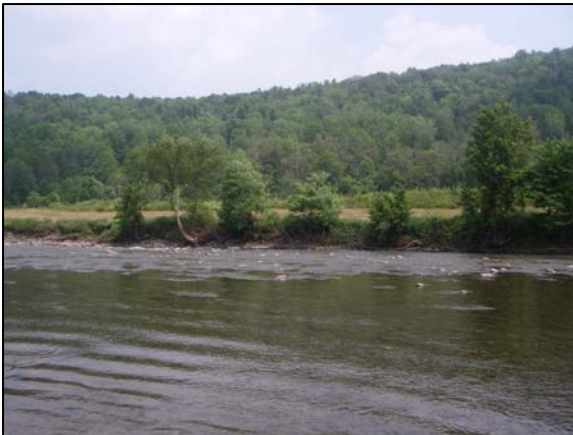
Bank erosion and planting site at Station 40300
