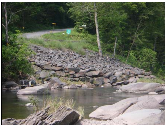
Rip-rap at Station 41200
