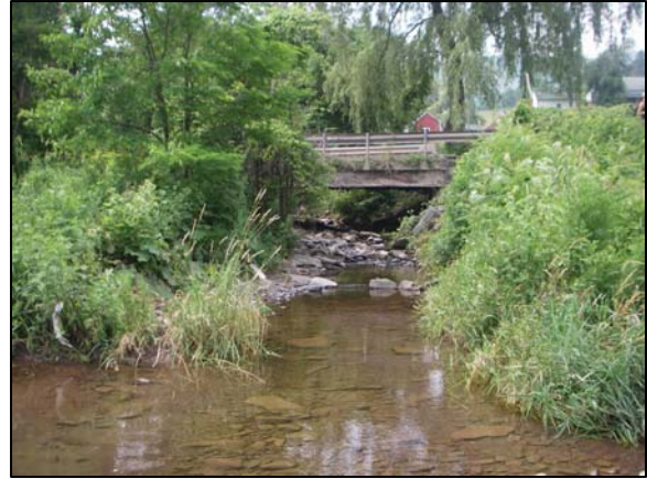
Tributary at Station 40300 - looking upstream
