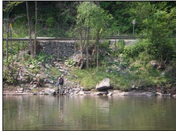
Little West Kill Road embankment
