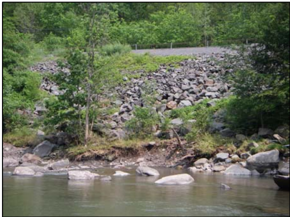
Rip-rap at Station 34050
