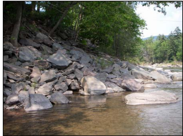
Rip-rap at Station 34360
