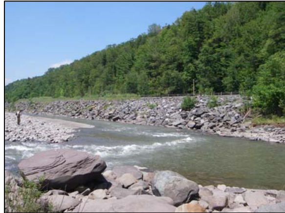
Rip-rap at Station 29750
