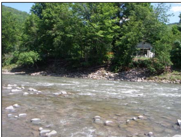
Bank erosion at Station 30600
