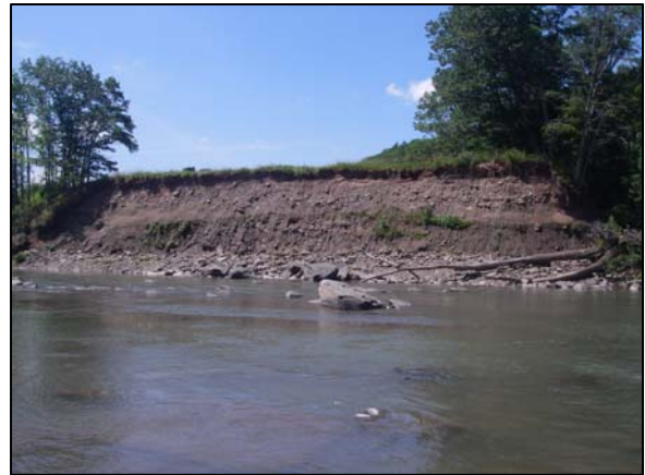
Bank erosion at Station 27950
