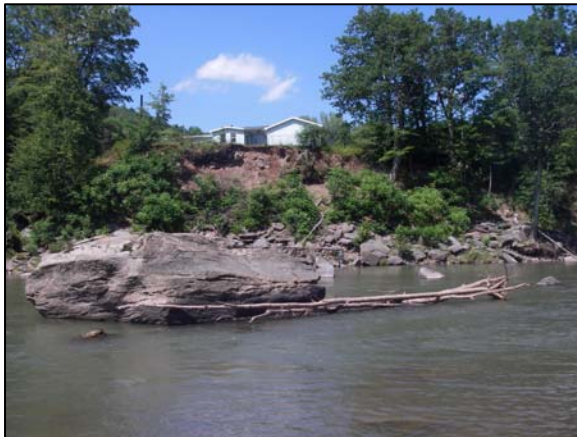
Bank erosion at Station 28100
