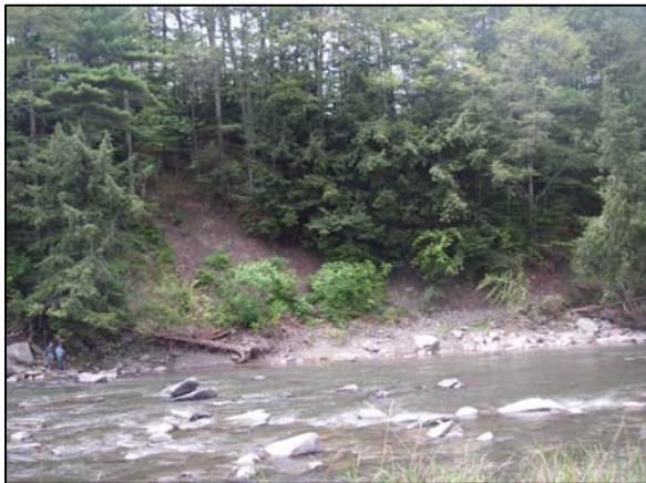
Bank erosion at Station 22800
