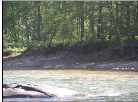
Bank erosion at Station 19100
