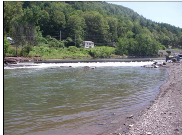
Dam at Station 15280 - looking upstream
