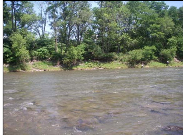
Bank erosion at Station 14400
