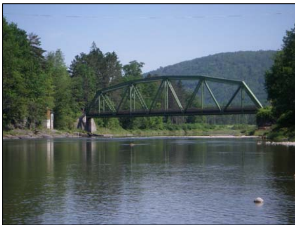
State Route 23 bridge in Prattsville - Station 10486
