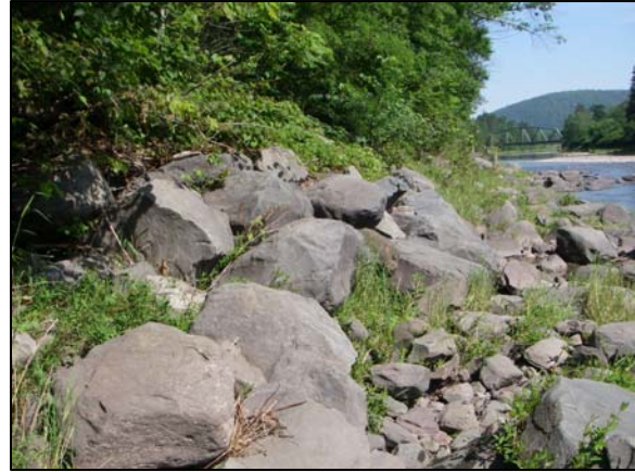
Rip-rap at Station 12100
