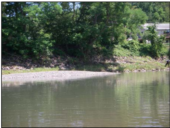
Rip-rap at Station 15150 - looking upstream
