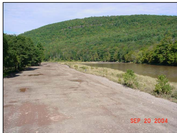
Prattsville flood redemption project post construction
