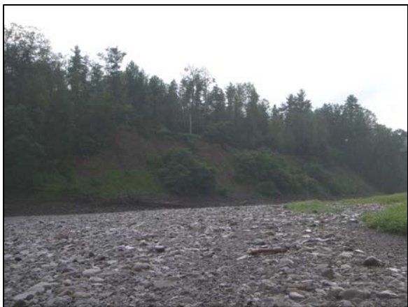
Bank erosion at Station 2250
