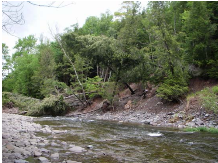
Photo 2.5.5. Hillslope failure in the Schoharie basin
