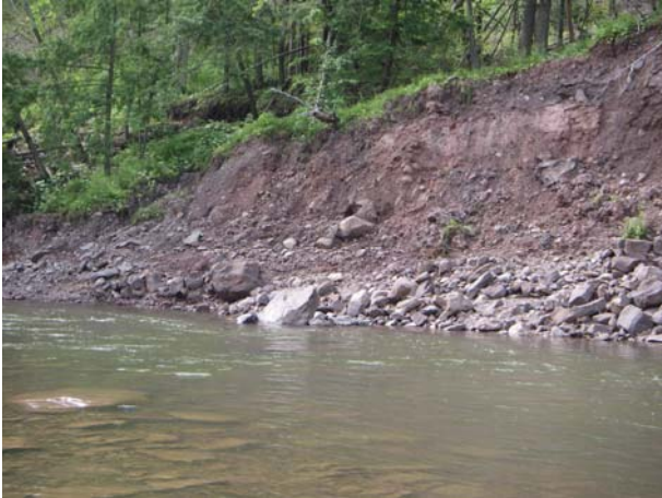
Glacial till with clay content exposed in streambank on Schoharie Creek
