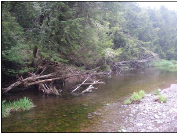
Bank erosion at Station 155250
