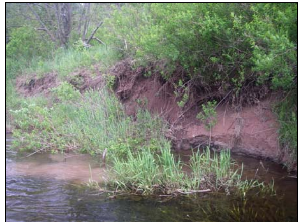
Clay exposure at Station 148740
