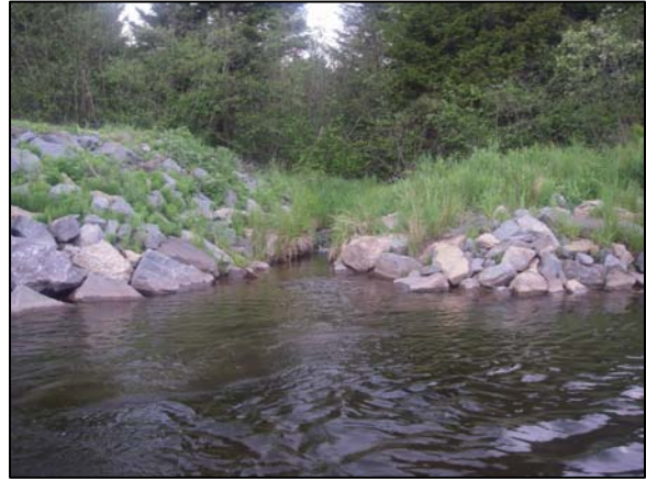
Tributary at Station 148690 - looking upstream
