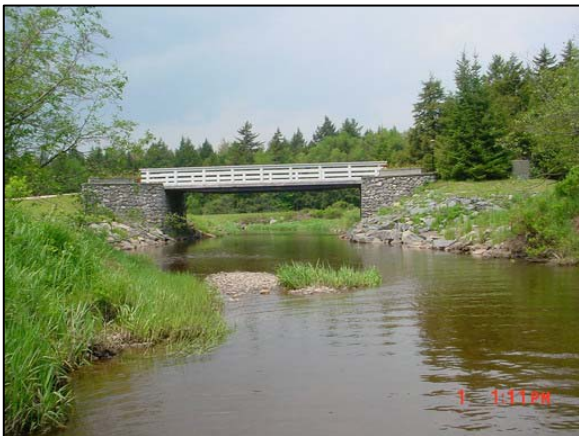
Bridge at Bunny Lane
