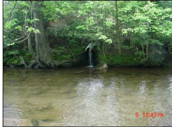
Piped outfall at Station 146830
