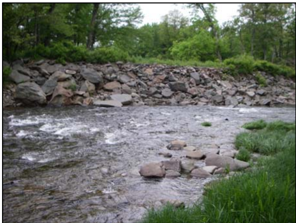
Rip-rap at Station 130850
