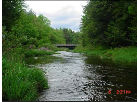
Bridge at Elka Park Road at Station 134100
