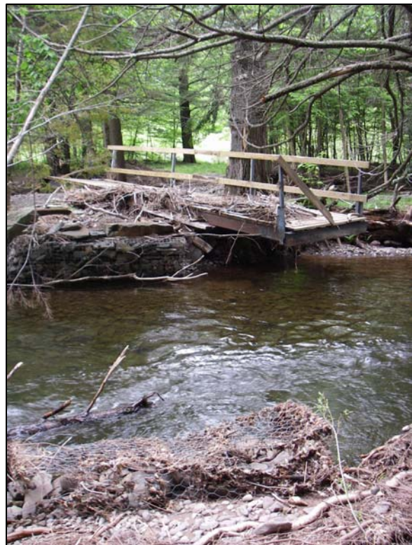
Bridge at Station 128070
