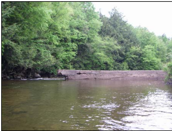
Dam remnants at Station 133700
