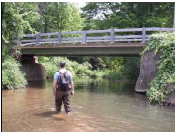
Champlin Road Bridge at Station 21930
