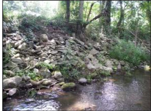
Revetment at Stations 22333
