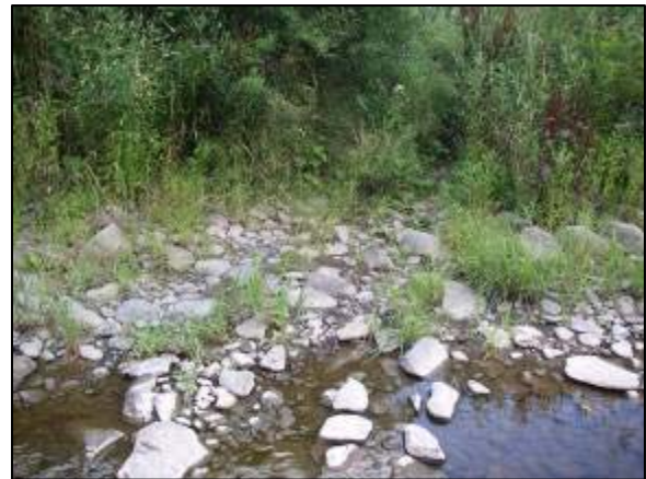
Channel Crossing at Station 19975
