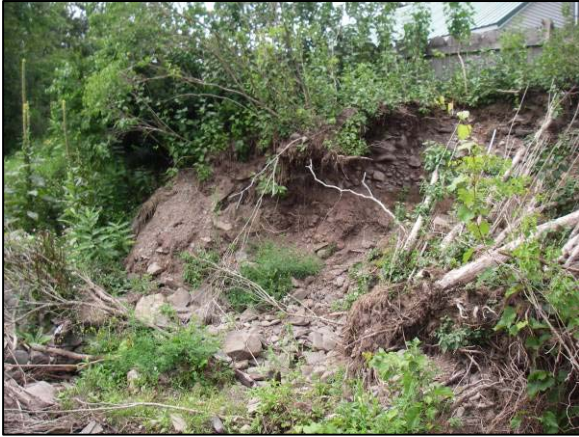
Erosion at Stations 17782 - 17690
