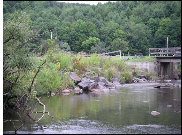
Revetment at Stations 16944 - 16874
