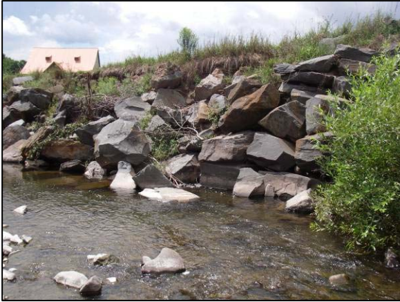
Revetment at Stations 17146 - 16971
