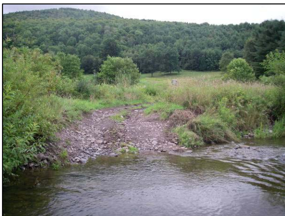
Channel Crossing at Station 16693
