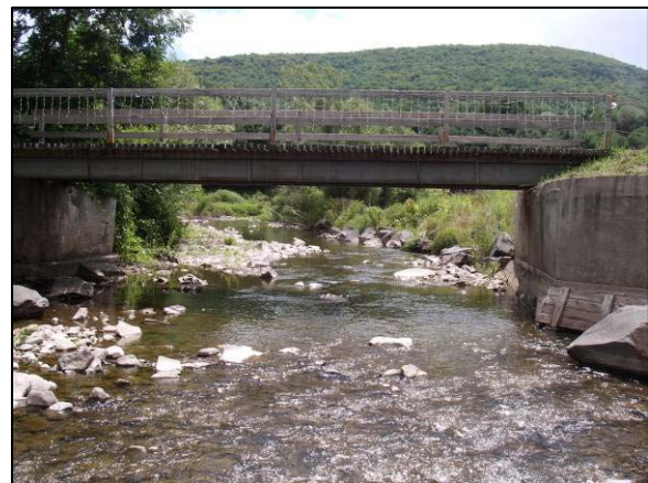
Bridge at Station 16957
