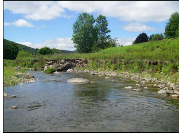
Erosion at Stations 15962 -15500 (downstream portion)
