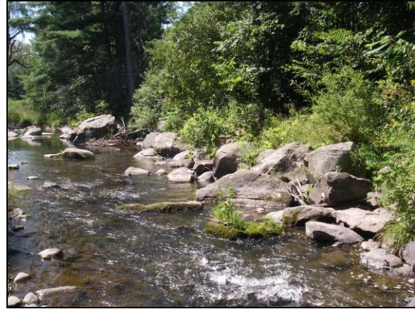
Revetment at Stations 9900-9779
