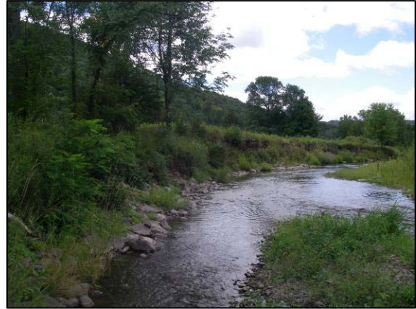
Erosion at Stations 15274 - 14944
