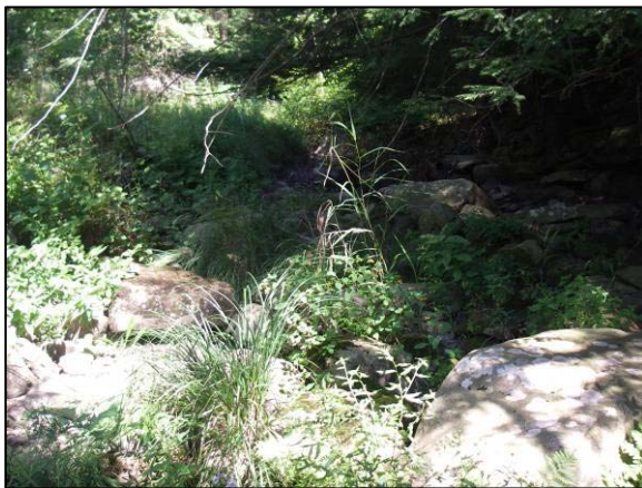
Flood Chute at Station 8426
