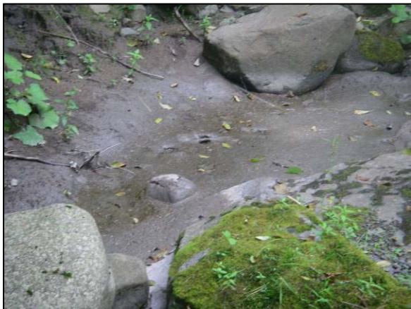
Clay Exposure at Station 6475
