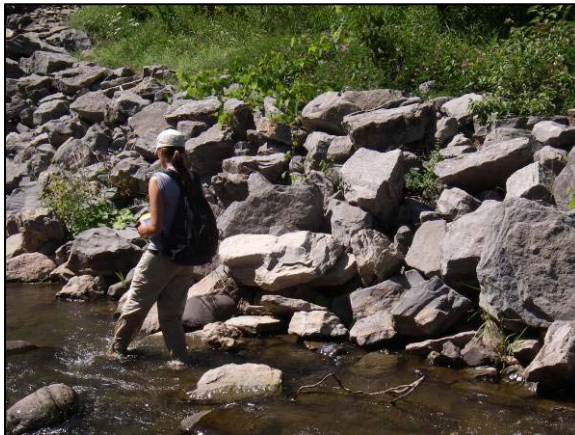
Revetment at Stations 8260-8165
