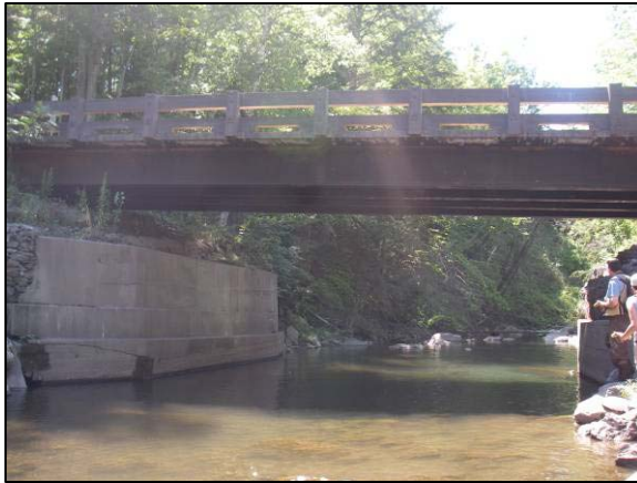
Bridge at Station 8167
