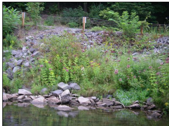
Revetment at Stations 7400-7367
