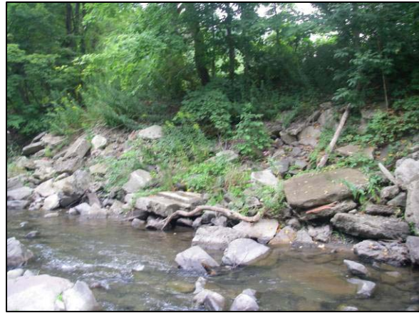
Revetment at Stations 7792-7657
