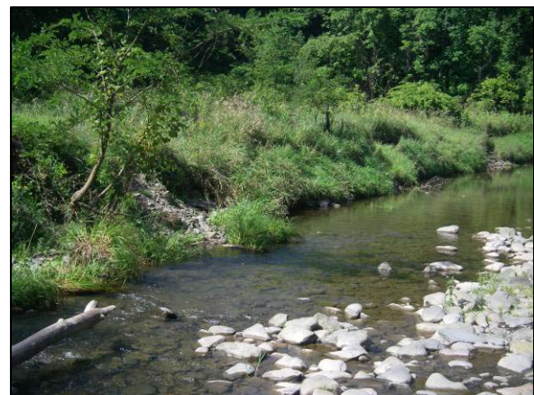
Erosion at Stations 2888-2552
