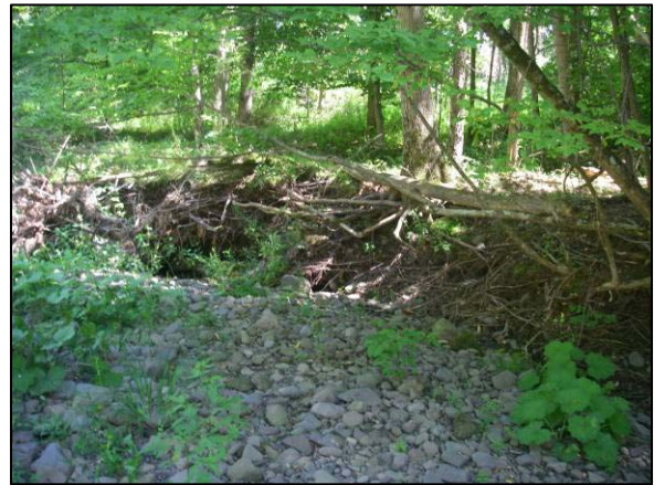
Erosion at Stations 1961-1891
