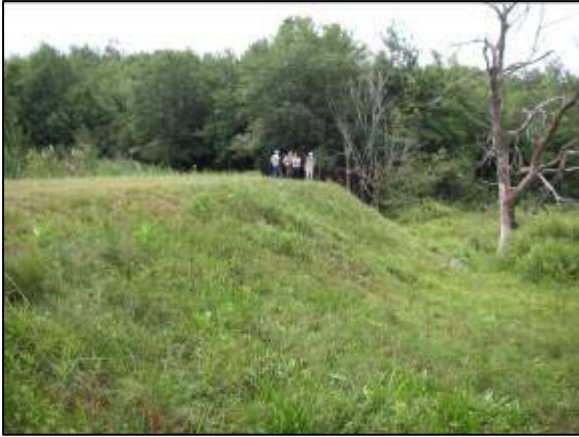
Private dam, Station 52058)
