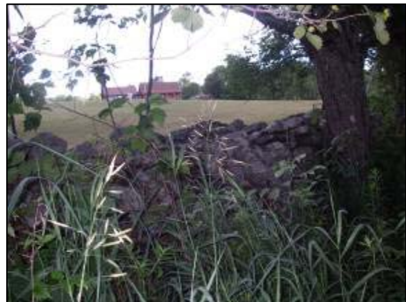
Berm at Stations 46900 - 46760
