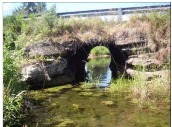
Culvert and Bridge at Station 45598
