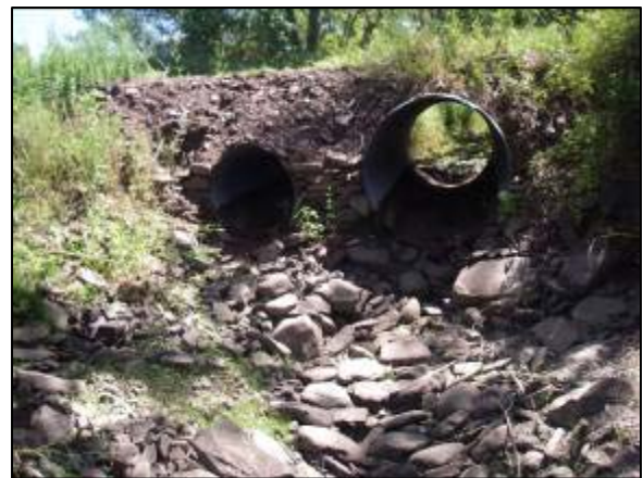
Bridge and Culverts at Station 46033 Photo looking upstream
