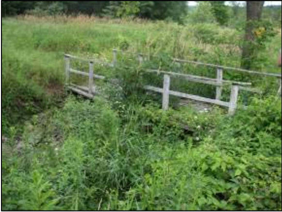
Bridge at Station 48807
