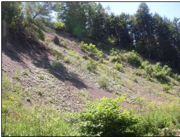
Mass Failure at Stations 40414 - 40265
