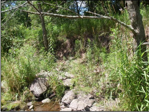
Erosion at Stations 44794 - 44741
