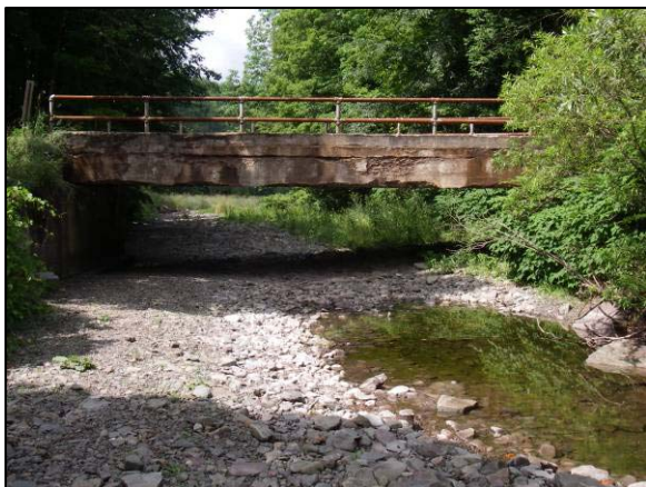
Bridge and Aggradation at Stations 38909 & 39020
