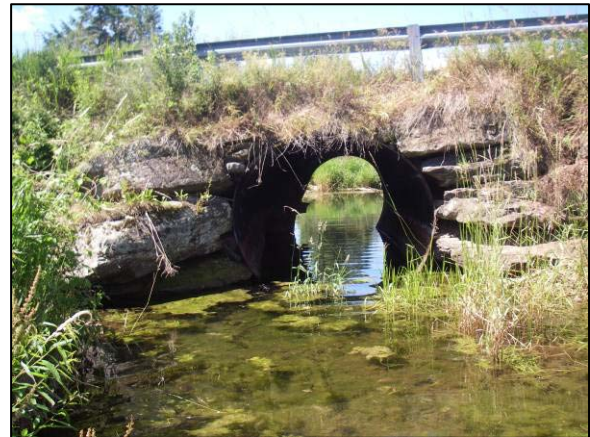
Culvert and Bridge at Station 45598
