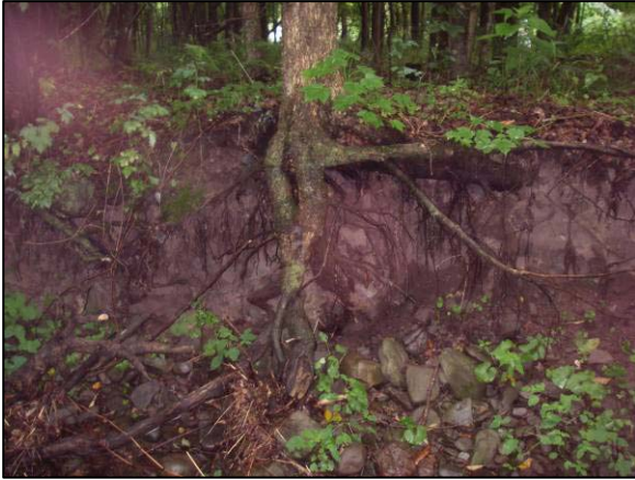
Erosion at Stations 39838 to 39801
