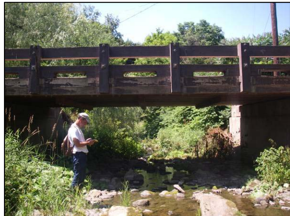
Bridge at Station 40631
