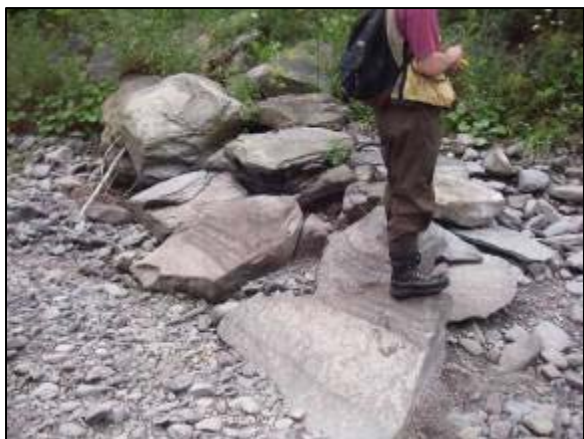
Rock vane at Station 38660
