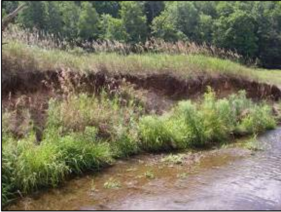
Erosion at Stations 31303 - 31180
