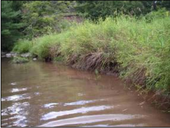
Erosion at Stations 27246 - 27183
