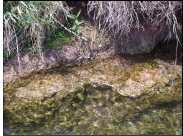
Clay Exposure at Station 33554
