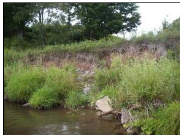
Erosion at Stations 28011 - 27857
