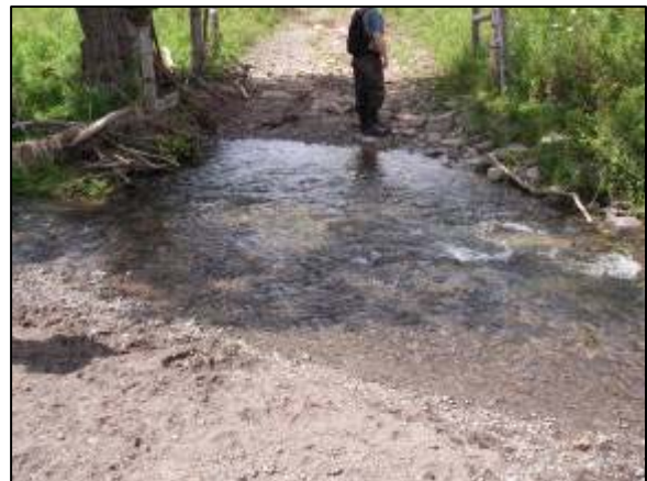
Channel Crossing at Station 28745
