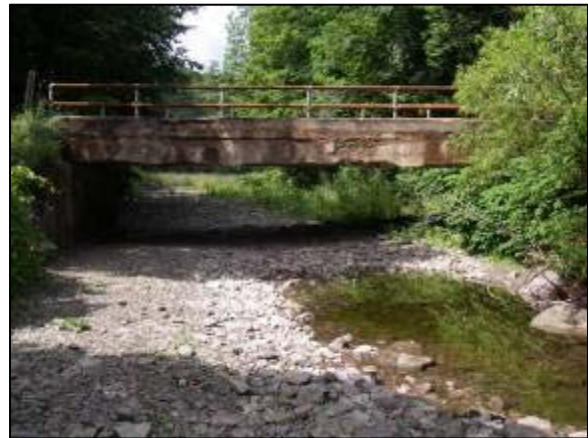
Bridge and Aggradation at Stations 38909 & 39020
