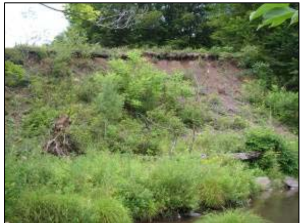
Mass Failure at Stations 27163 - 26938
