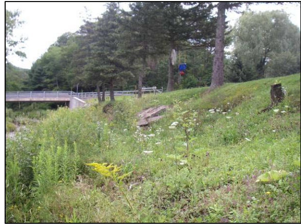
Riparian Planting Site at Stations 25833 - 25673
