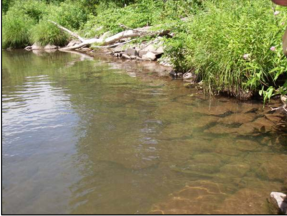
Revetment at Stations 26750 - 26712
