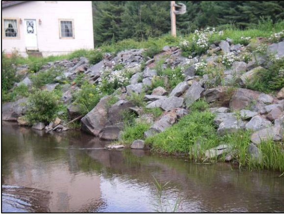
Rip rap at Stations 25485 - 25301
