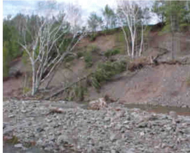
Figure IV-32: Under conditions of extreme stream instability, riparian vegetation can be ineffective in providing streambank stability as shown in this eroded terrace in Big Hollow.
