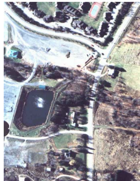
Figure IV-45: Aerial view of stormwater treatment pond at Ski Windham. The pond captures runoff and provides a controlled release to the stream system.
