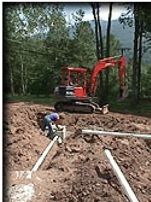
Figure IV-44: Replacement or upgrades of failing septic systems is a high priority of NYCDEP and the Catskill Watershed Corporation. (CWC)
