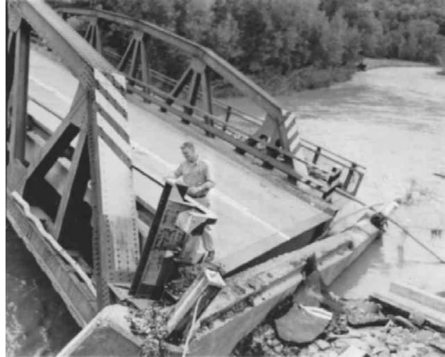
Figure IV-46: Bridges over the Batavia Kill or the tributaries have often been the subject of extensive damage due to flooding.
