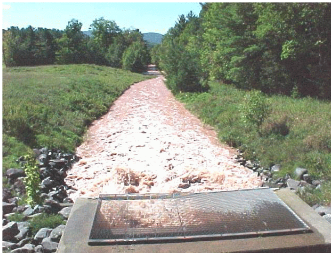
Figure V-24: Discharge from the C.D.Lane dam spillway 2 days after tropical Storm Floyd.
