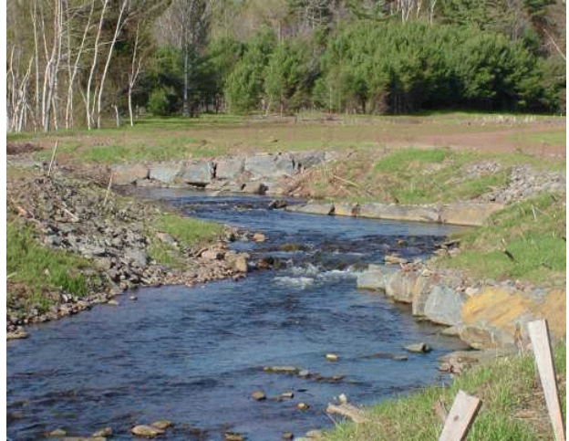
Figure VI-9: View of restoration work undertaken in segment 1c during 2001.
