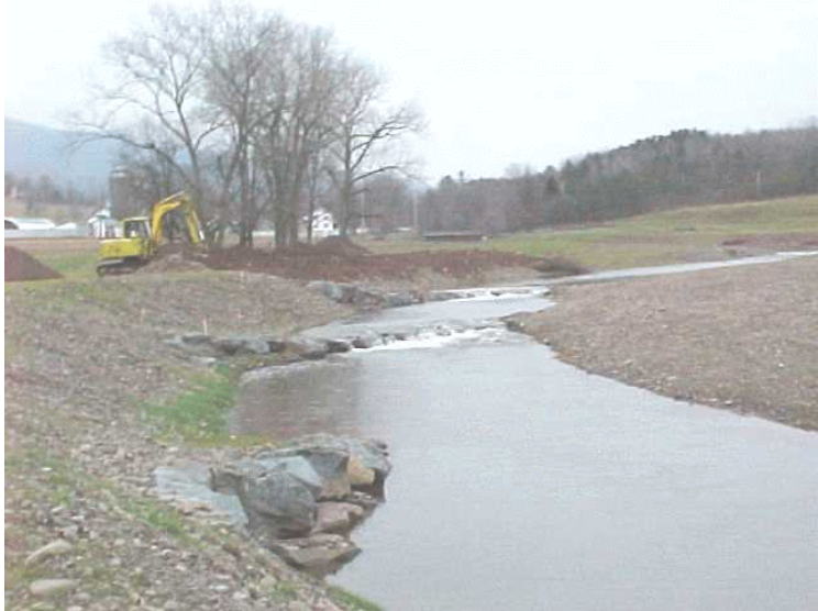
Figure III-23: View, looking upstream, of 3 rock vanes. Note that water is deflected away from the streambank.
