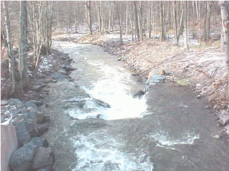
Figure III-24: View of a cross vane from upstream. Note that velocities are placed in the center of the stream channel and still, flat water is located along the banks upstream of the structure.
