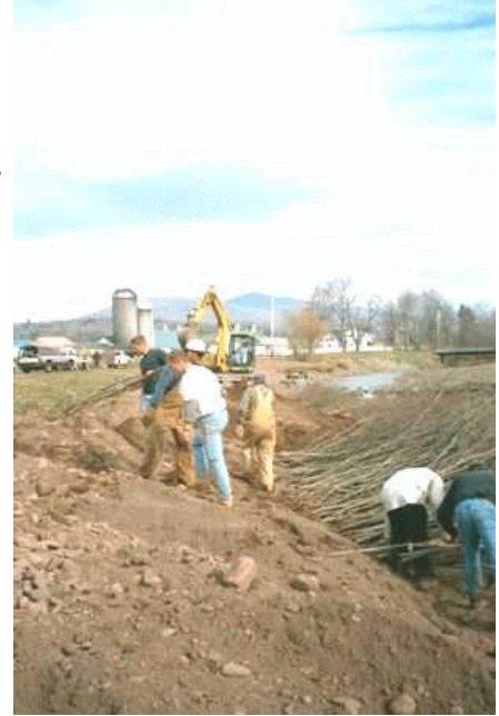
Figure III-25: Installing Brush Layering.
