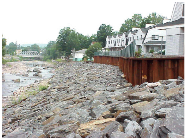
Figure III-21: Hardened streambanks can transfer erosional problems downstream.
