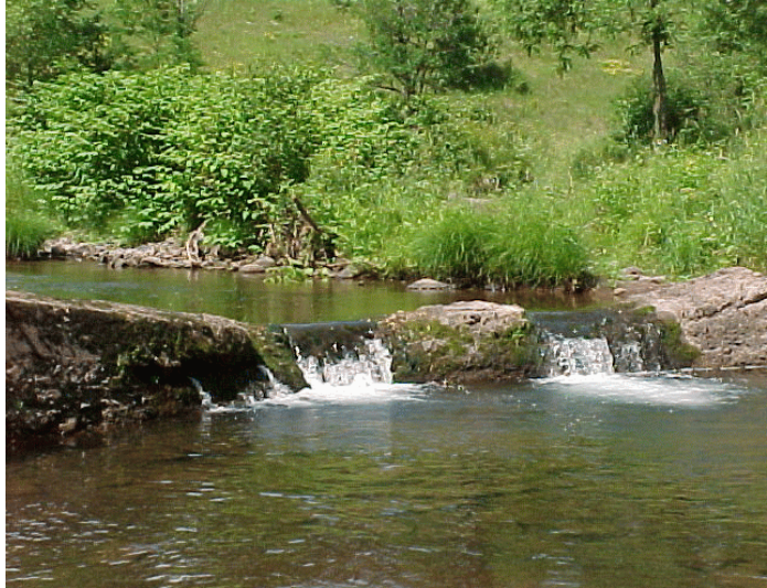
Figure III-20: Old concrete check dam on the Batavia Kill.
