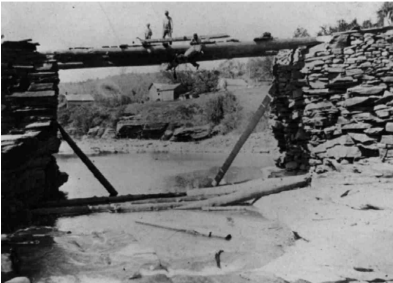
Figure IV-3: Maintaining the bridge at Red Falls, circa 1910. Photo by Everett Arnold Conine.
