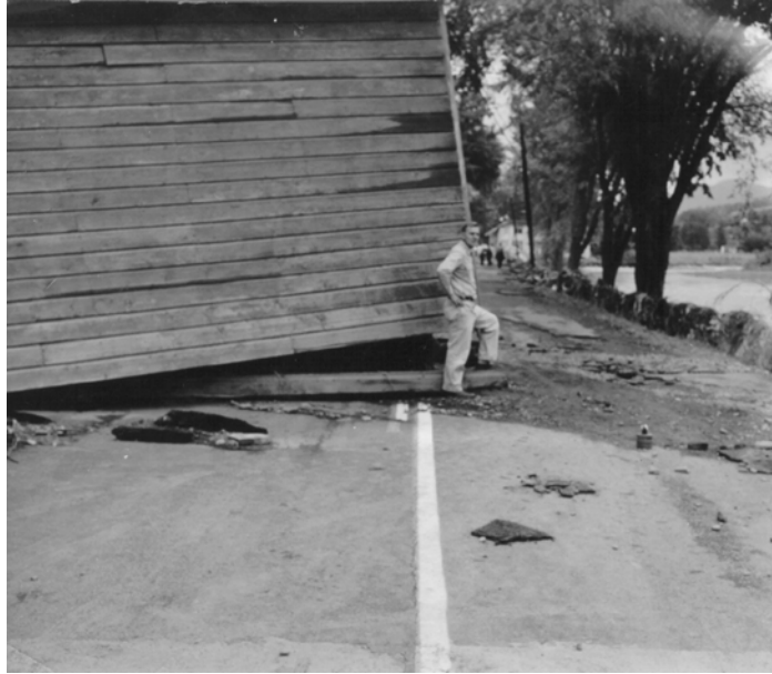
Figure IV-5: Flood damage to barn along NYS Route 23 circa 1961.
