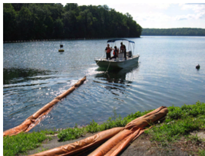
Figure 3.3 Wave stabilization boom installation.
