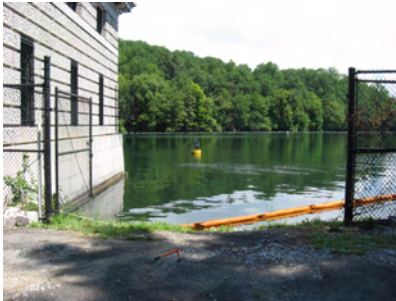
Figure 3.4 Wave stabilization boom connection to the Catskill Upper Effluent Chamber.
