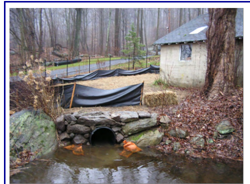
Figure 5.1 Remediation of an eroded watercourse in the East of Hudson watershed.
