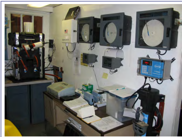
Figure 1.6 Continuously recording equipment used to monitor water quality in the aqueducts.
