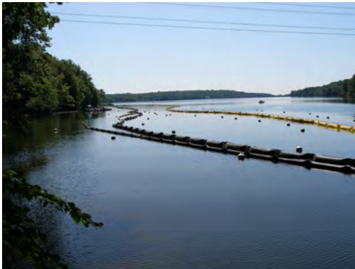
Figure 3.18 Turbidity curtain in Ken-sico Reservoir at the Catskill Upper Effluent Chamber (UEC) diverts stormwater away from the intake.
